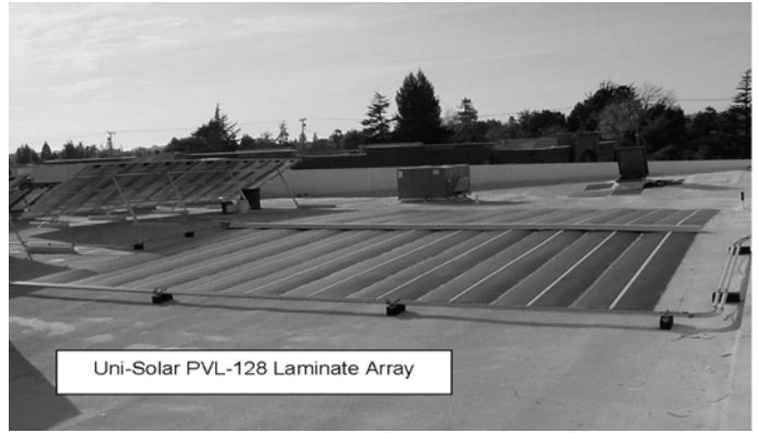
Figure 4 Santa Cruz Site: Laminates mounted horizontally
